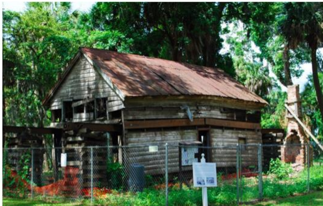
Figure 3.4 Failed Stabilization at Garvin House This image shows the Garvin House after the cribbing failed, c. 2012. Image courtesy of Erin Schumacher
